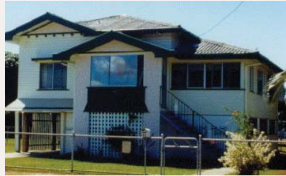
Hip and gable, VJ lining, reduced rafter spans, on stumps (low and high)
