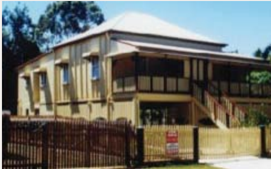
Hip roof, reduced rafter spans, central core, exposed studs, on stumps (low and high)
